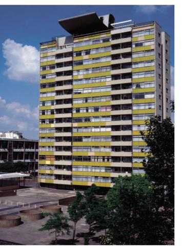
Figure 2.26 Golden Lane tower clad in yellow curtain walling.
